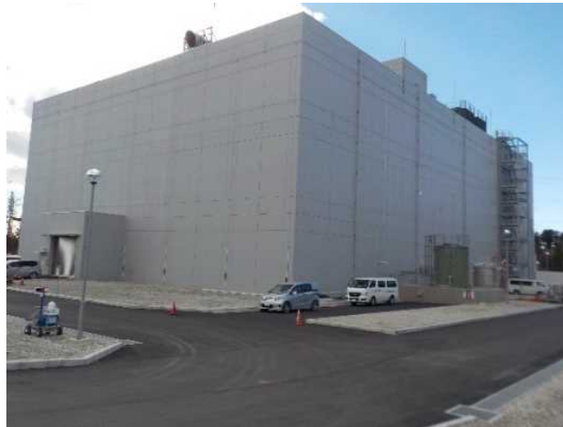
Miscellaneous solid waste incineration system building
