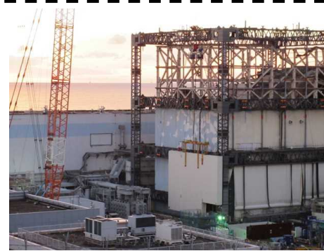
Removal of panels (Nov, 2016)
