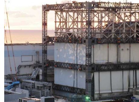
Complete removal (Nov, 2016)
