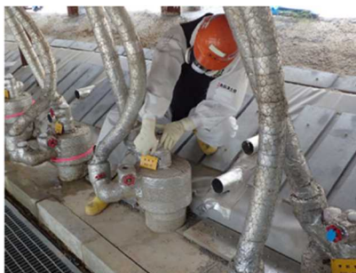
Opening a valve on a freezing pipe (Phase 2)
