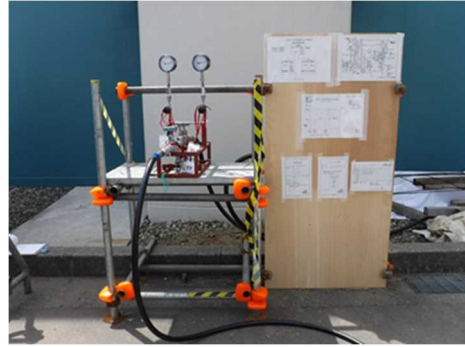
Pressure testing of pipes (Unit 6)
