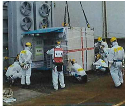
Installation of measurement device
