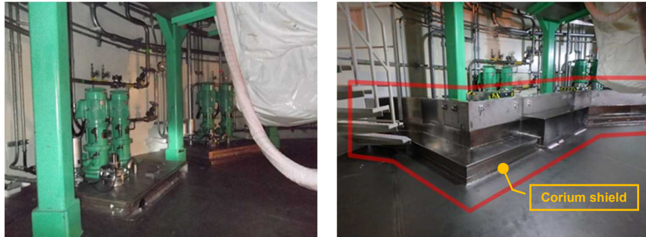
Installed corium shield (Unit 7) (Left: before; right: after)
