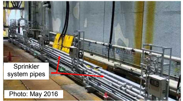
Installation of sprinkler system pipes
