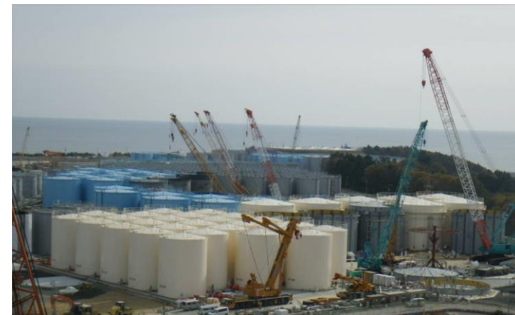
Tank construction and removal progress report
