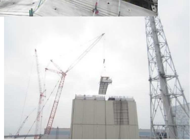
Removal of roof panel
