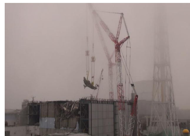
Removal of refueling equipment
