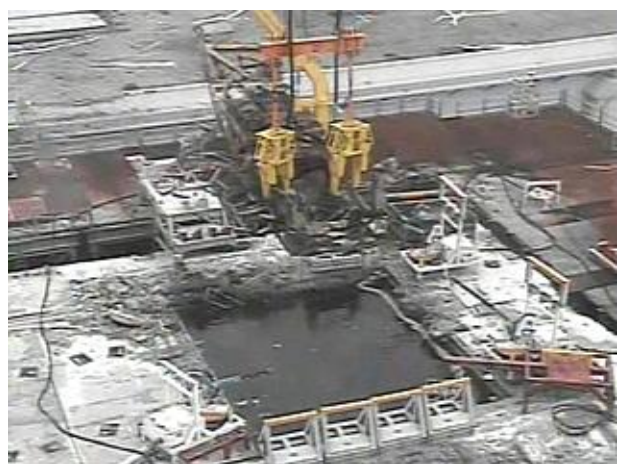
Removal of refueling equipment
