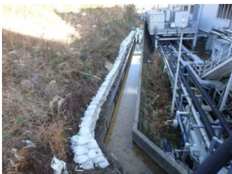
Cleaning of side ditch that leads to drainage channel K
