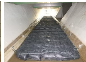
Cleaning of drainage channel K and installation of purification material
