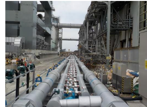
Situation of installation of cooling pipes
