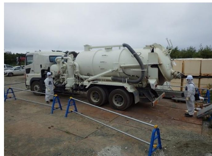
Arrangement of personnel during operation of tank cover
