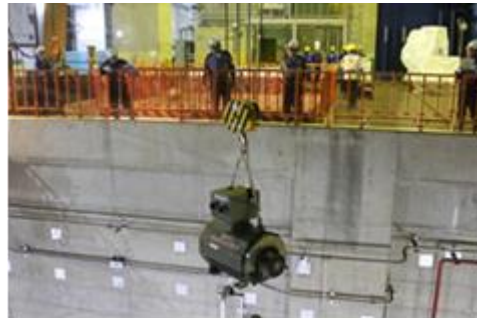
Motor replacement (transporting spare motors)
