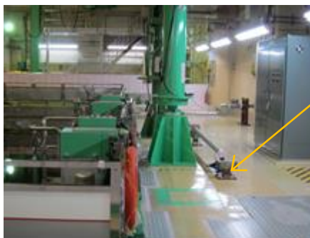
Installation of spray piping from the outside of the building to the spent fuel pools (Unit 2)
