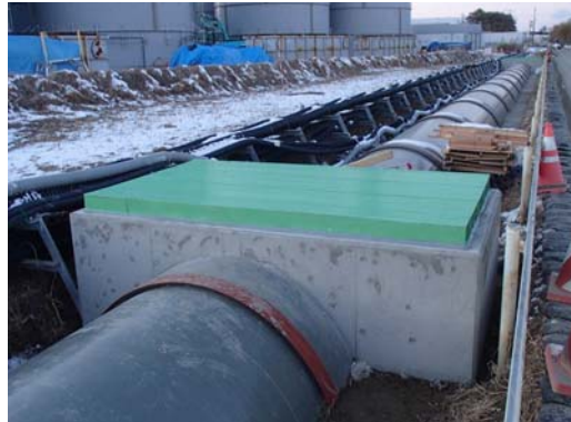
Situation of the B-drainage channel with culvert
