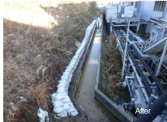
Situation of cleaning the side drain at the K-drainage channel
