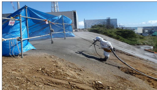
Situation of spraying on the sloped surface
