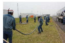
✓ Trainings to connect temporary cables
