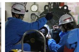
✓ Trainings to restore cooling water pumps
