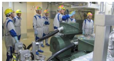
✓ Power station safety inspection undertaken by executives
