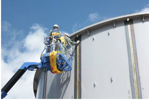
Welded part inspection
