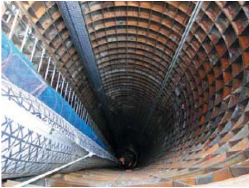
Shaft for fault investigation 30m underground
