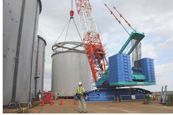
Large crane lifting a tank to load on a transport boat
