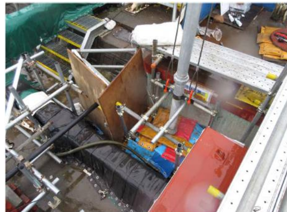
Loading blocking material at Unit 2 seawater piping trench tunnel
