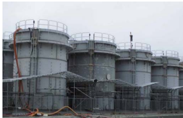
Improvement-2: Flange type tanks after installation of weir covers
