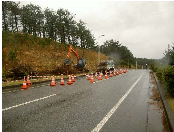
Installation of a firebreak
