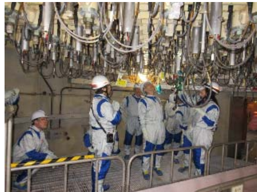
Beneath a nuclear reactor (pedestal) (Unit 4)
