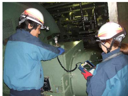
Vibration check for shaft bearing of rotating equipment
