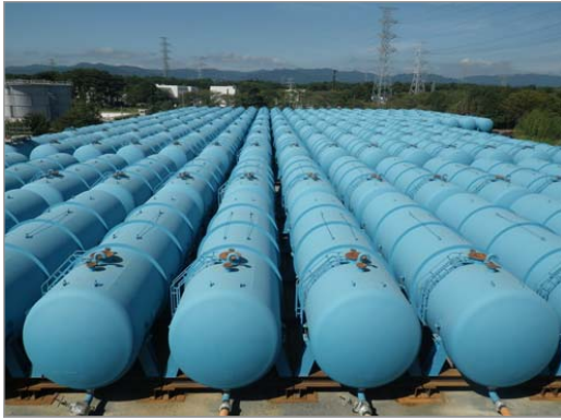
Improvement-1: Tank placement in H1 area before improvement
