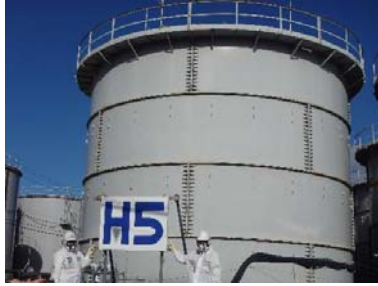
Identification board in tank area (Fukushima Daiichi)
