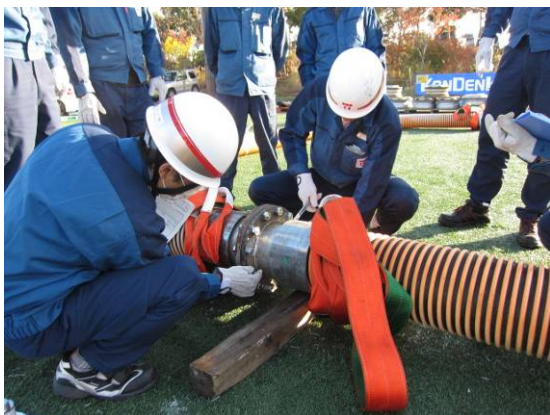
Temporary hose (Kanaflex) connection drill at Fukushima Daiichi (Left: Hose to hose connection, Right: Connection to different diameter flange)
