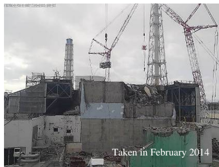
After Debris removal
