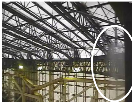
Spraying of anti-scattering agent
