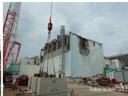
After Debris removal
