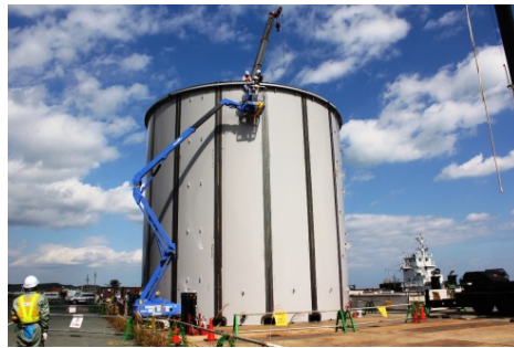
Tank manufacturing at Fukushima Daiini
