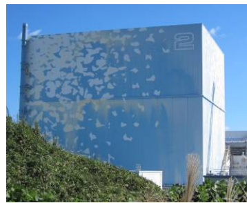
Unit 2 Reactor Building
