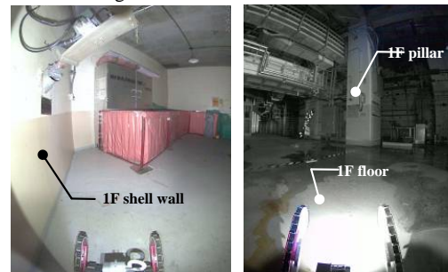
Reactor Building framework survey
