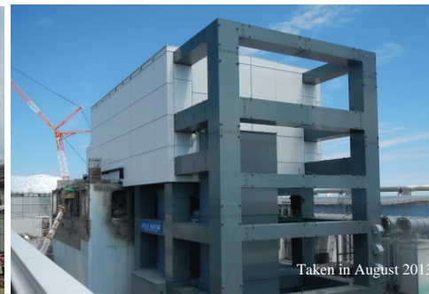
After Fuel removal cover installation
