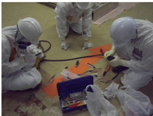
Training for handling low-tension cable terminals
