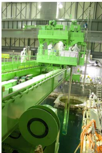
Status of fuel removal
