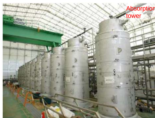
Installation of high-performance multi-nuclide removal equipment
