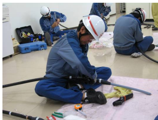
Training for handling high-tension cable terminals
