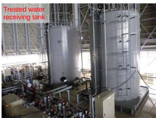
Installation of extended multi-nuclide removal equipment
