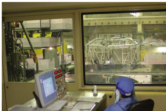
Monitoring operator to check entire status from the operation room of the fuel handling machine
