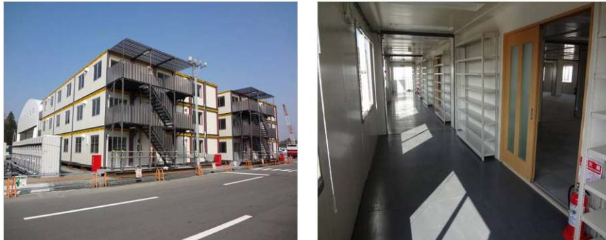
Temporary ex-site rest station (External view / Inside)
