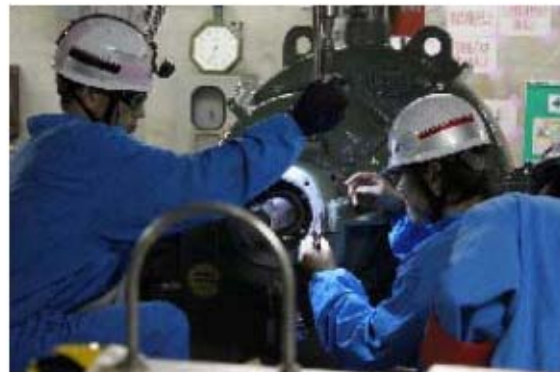
Cooling Water Pump Restoration training (bearing assembly)
