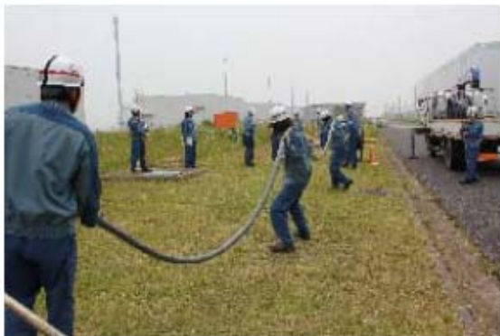
Temporary cable connection training (Cable installation)
