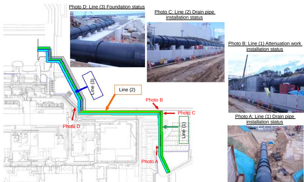
Work progress to switch discharge channel route
