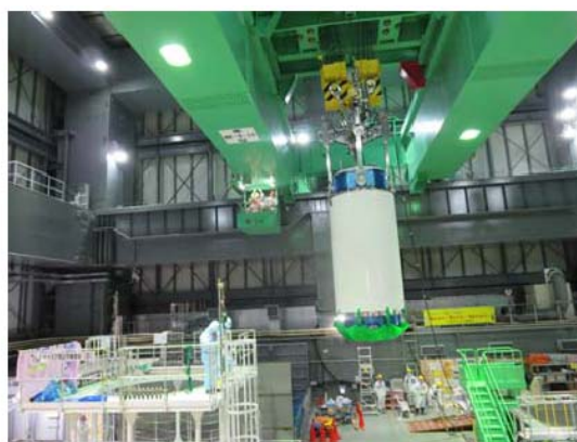
Transfer of spent fuel transportation container
