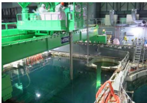
Fuel removal from spent fuel pool
