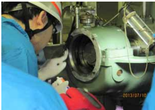
Work restoring a cooling pump
