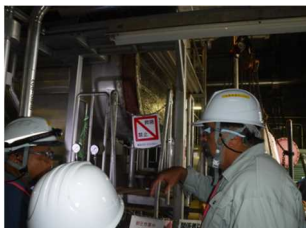
Field inspection by NSAB members (Fukushima Daiichi)
