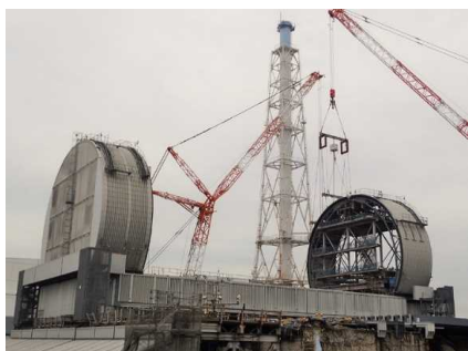
Unit 3 Fuel removal cover (dome roof) installation (September 6)
