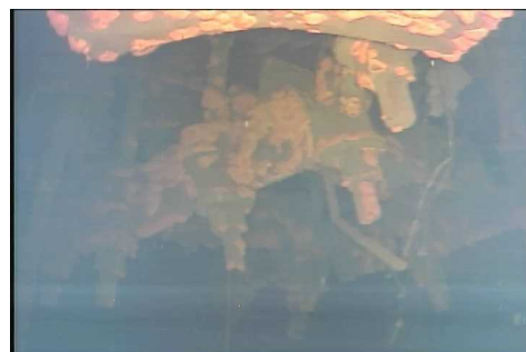
Survey of the bottom of the Unit 3 PCV (July 19) [Support structure for control rod drive mechanism]
