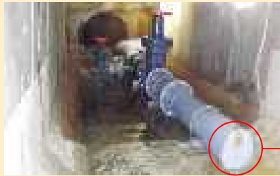
Installed check valve
