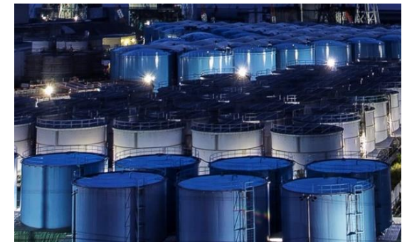
Treated water storage tanks
