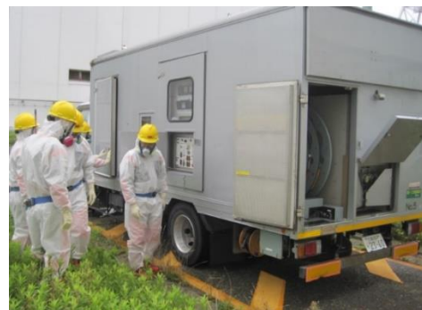
Repairing power source in radiation protection gear
