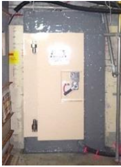
Opening after sealing
