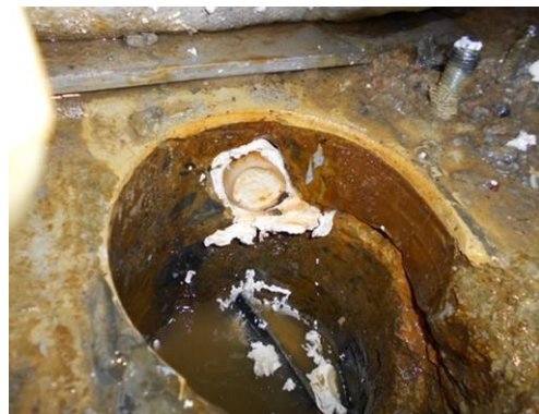
Floor funnel sealed using filler material
