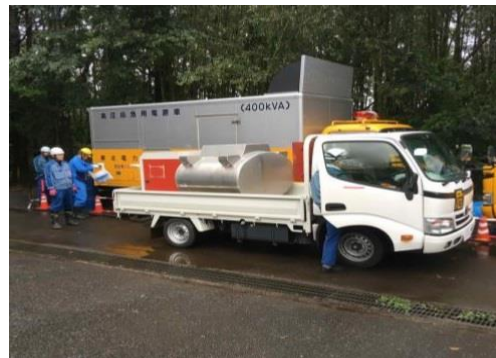
Filling a power supply truck with gasoline using a tanker truck from Fukushima Daini
