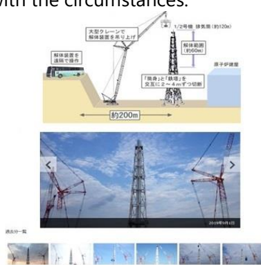
Unit 1/2 exhaust stack dismantling page
