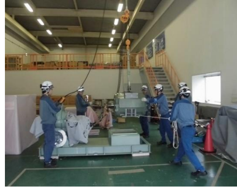
Generator replacement training
