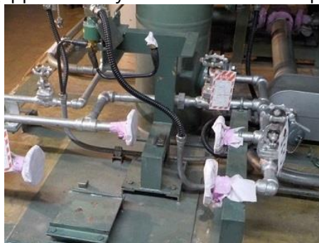
Prior to kaizen: Covered with fire-proof sheet
