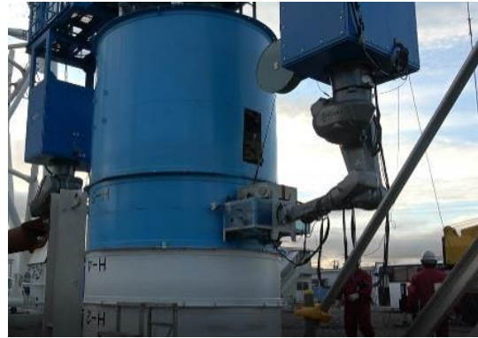
Cutting around the circumference of the stack
