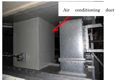
After air conditioning duct installation
