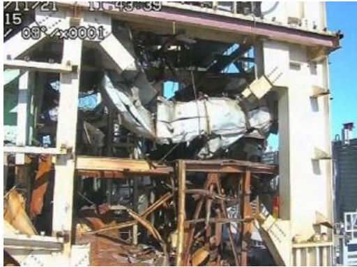
Left: After removal of X-brace on south side
