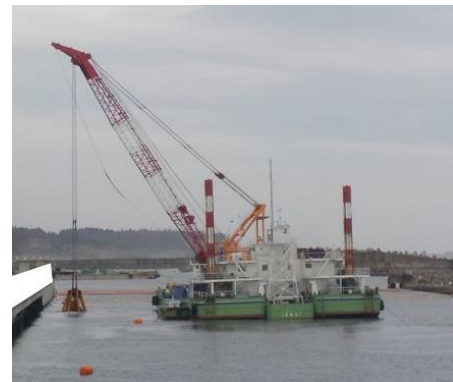
Open water construction
