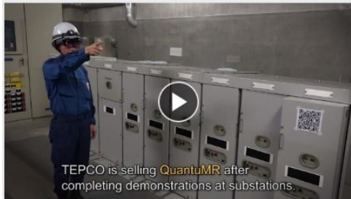
Facebook post on QuantuMR that was announced at the end of November Tokyo Electric Power Company Holdings, Incorporated: Using MR to support field work... We have launched our #QuantuMR system together with Pocket Queries. This system uses Mixed Reality technology to provide operational and safety support with a remote communication function. An overview of QuantuMR can be viewed here : https://mz-...
