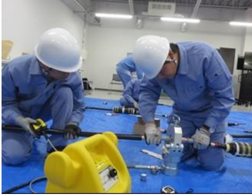
High-voltage cable terminal preparation/connection training
