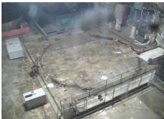
Operating floor (after clean-up)
