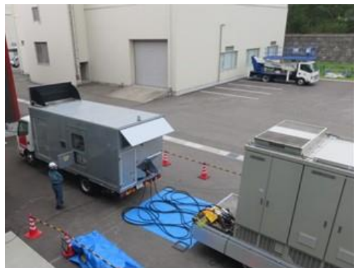
Power supply truck operation training (High-voltage e load truck connection)
