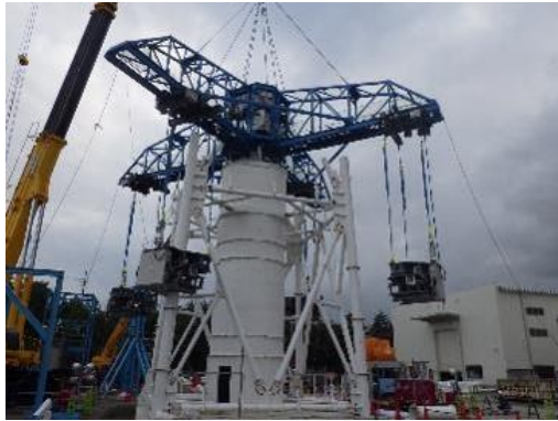
Dismantling the main pillar
