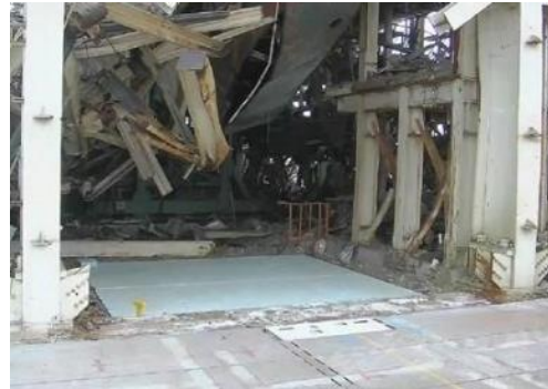
After covering opening (equipment hatch)
