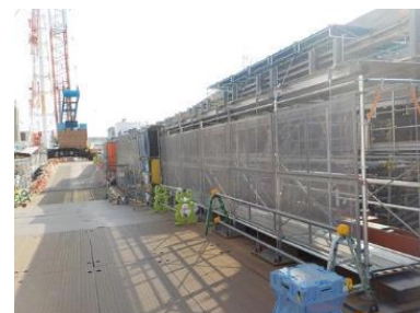
Roofed safety passage
