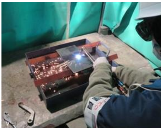
Welding/cutting/grinding (gas torch cutting)
