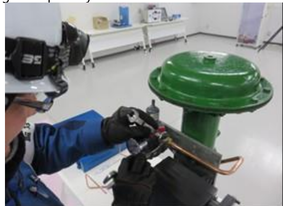
Valve/drive mechanism (AO copper pipe fitting) training
