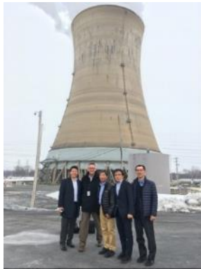
Three Mile Island Nuclear Generating Station
