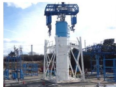
Dismantling exhaust stack mock-up
