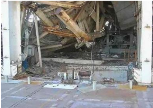
Prior to covering opening (equipment hatch)
