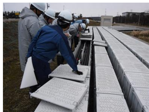
Cable splicing investigation
