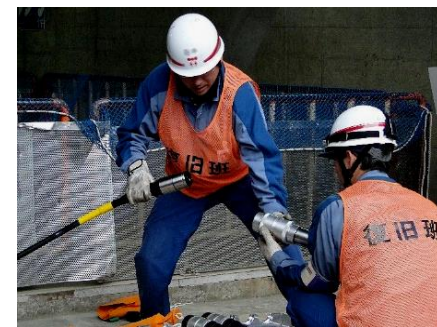
Training on connecting cables to power supply trucks
