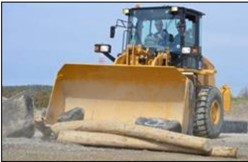
Removing debris using wheel loaders
