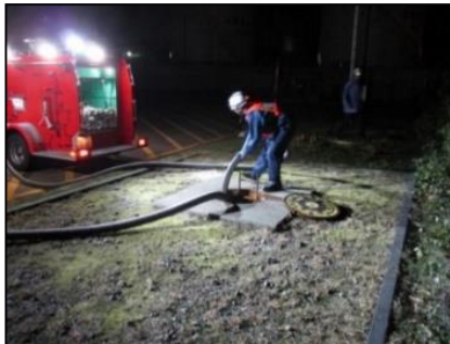
Injecting cooling water using fire trucks
