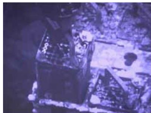
Fuel removal work
