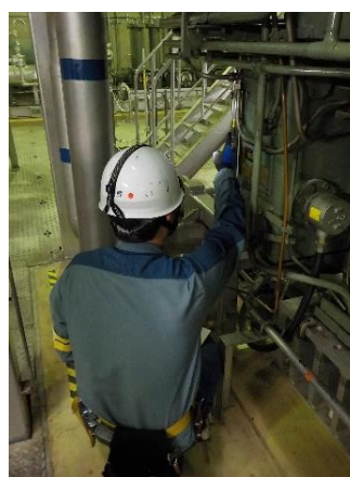
Changing lubricating oil tank refueling procedures to reduce the risk of oil leaks (Kashiwazaki-Kariwa) Right: Opening tank refueling valves Left: Checking tank refueling levels
