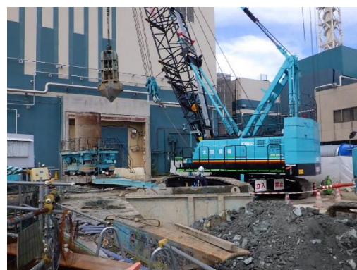
Ground improvements for the large freight entrance
