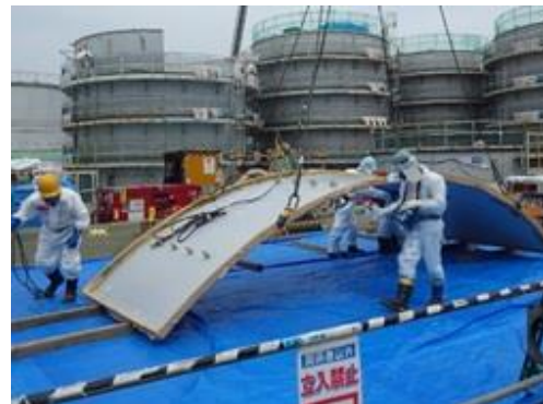
Flanged tank dismantling kaizen (Fukushima Daiichi)
