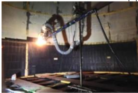
Flanged tank dismantling kaizen (Fukushima Daiichi)
