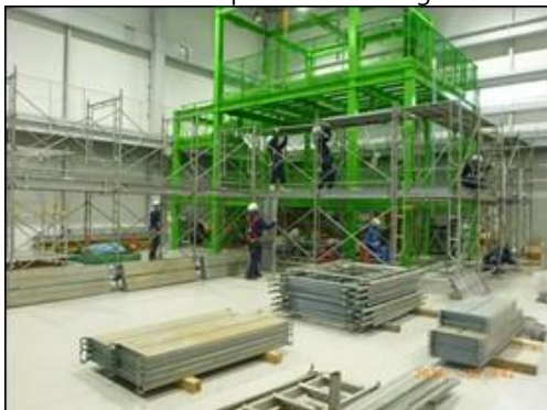
Scaffolding assembly training
