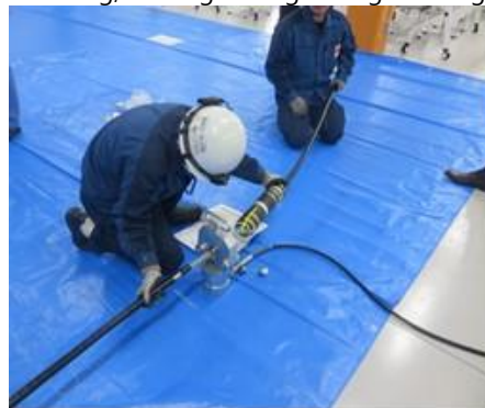
Cable terminal preparation/connection training
