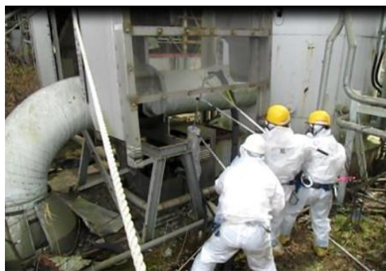
Suction pipe replacement
