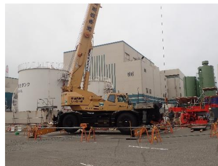
Unit 6 diesel fuel tank
