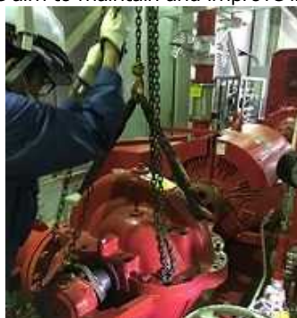
Fire pump repair training (hoisting)
