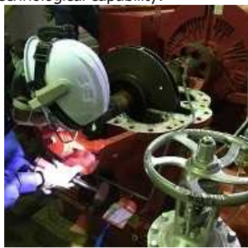
Fire pump repair training (overhaul)
