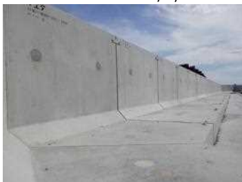
Kuril-Kamchatka Trench Tsunami Seawall
