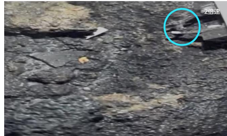
Photo taken in October 2024 Unit 2: End jig grasping fuel debris
