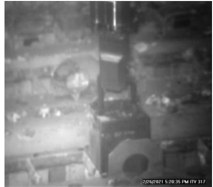
Lifting up fuel in Unit 3 (568 fuel assemblies)
