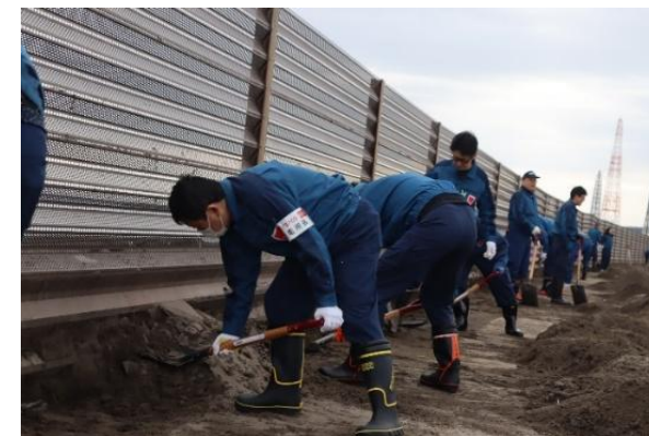
Coastal sand removal
