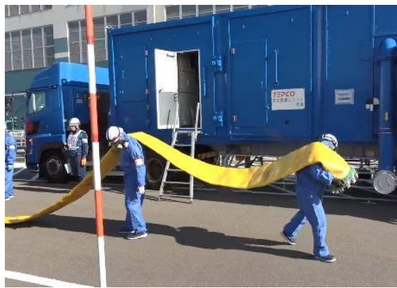
Training on connecting substitute heat exchangers
