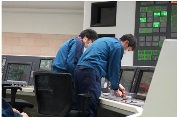
January 21 reactor startup
