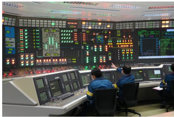
February 16 Commencement of power generation
